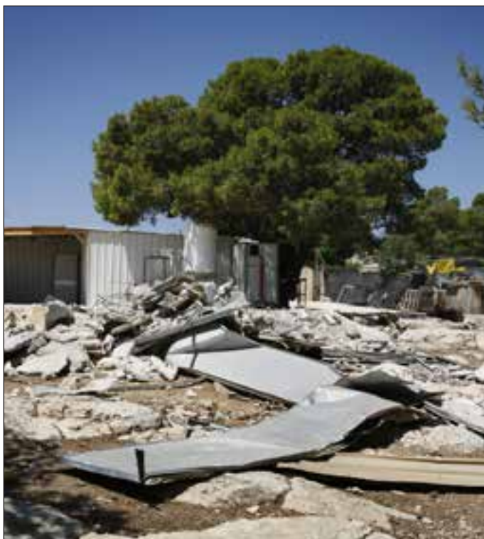
Demolished Palestinian structure in the West Bank. Israel routinely destroys Palestinian homes and buildings, including infrastructure build by the EU.
