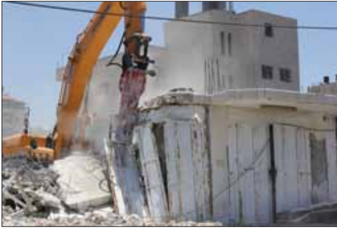
Shops and homes being demolished in Beit Hanina
