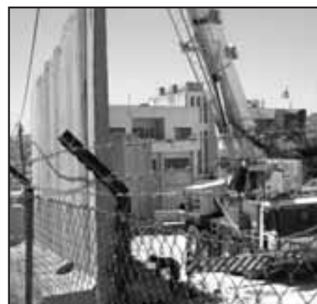
The Wall being built around Bethlehem, separating Palestinians from Palestinians
